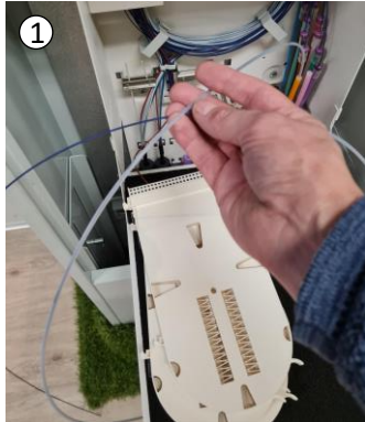
① Push a predefined length of 3mm tube onto the Stingray unit
