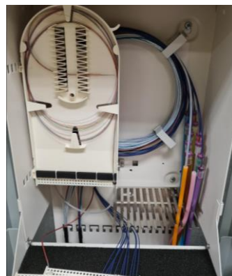
⑤ Route the fibers in the protection tube the desired way towards the splice cassette
