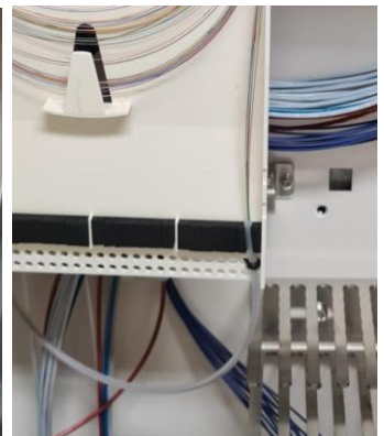
⑤ Route the fibers in the protection tube the desired way towards the splice cassette
