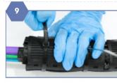
9 Fix the cable ties in the position shown to ensure sealing. Start fixing the ties from center position and then outwards in both directions. Cut the excess cable tie length.
