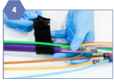
4 Wrap the MTPPE tapes around the ducts with contours on the outside.
