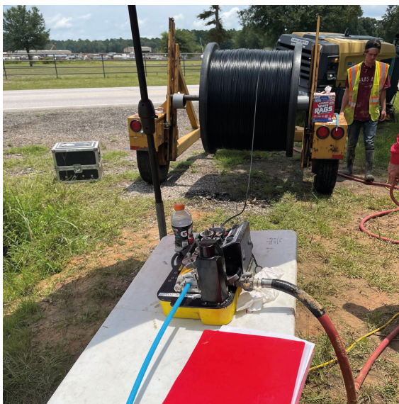
A high-powered air compressor blows the micro fiber cables through the microducts at speeds of 500' per minute.
